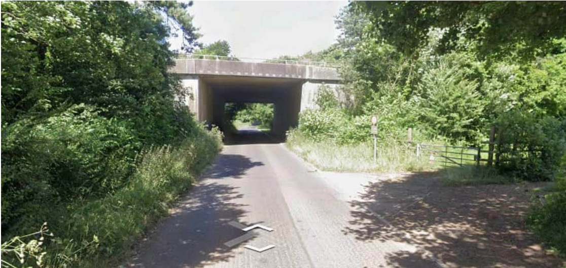
M4 Overbridge at Littleton Drew 18ft maximum clearance
