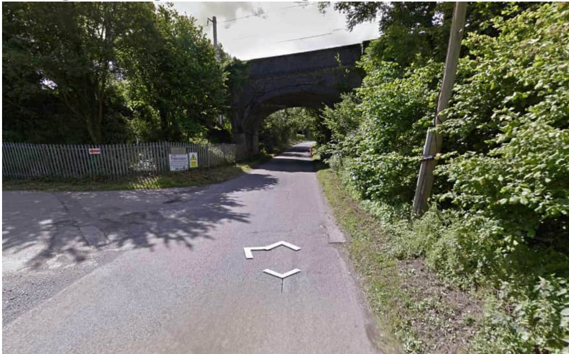
Fosse Way rail bridge (restrictions unknown)
